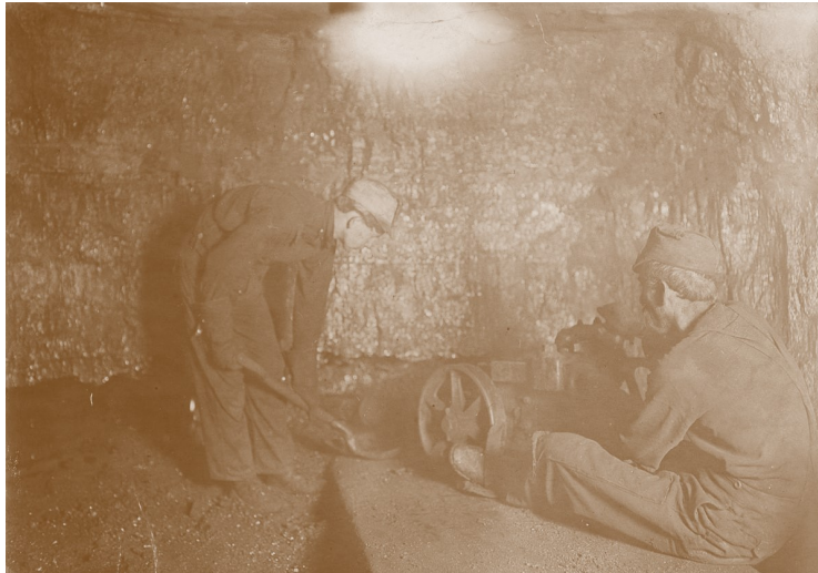
Boy Shovels Loose Coal at Laura Mine, Red Star, W.Va.
